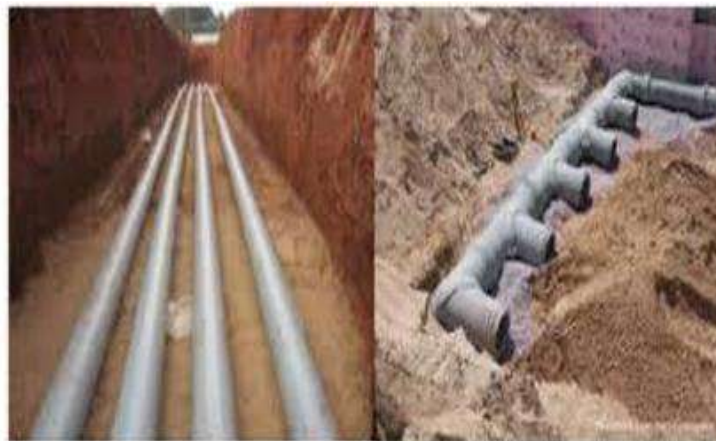
Figure: 1 EAHE setup of PVC material.
